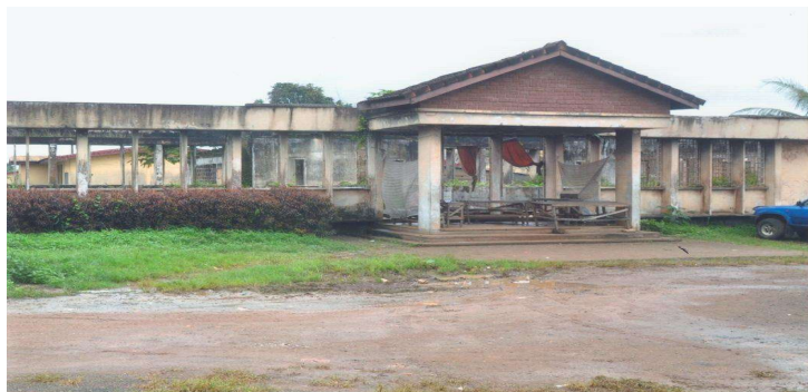
Figure 1.2 Destroyed Taxation Centre Meme, Kumba
